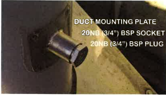
101: Flow Measuring Port Detail
